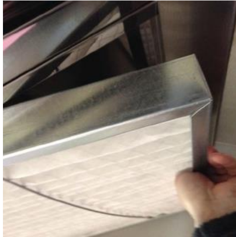
Stage 2 Filter Panel Replaced
