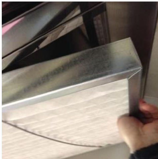
Removing the Stage 2 filter
