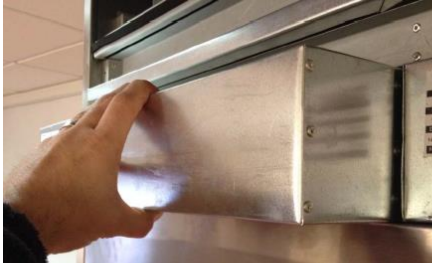
Sliding the Stage 3 Filter Panel Forward
