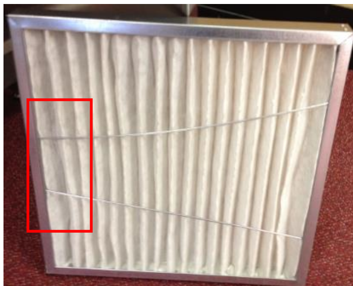
Replacing the Securing Clip over the Stage 2 Filter Pad
