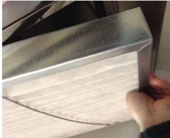
Removing the Stage 2 filter
